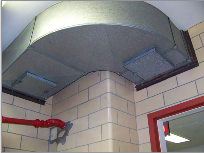
Ductwork that does not serve the stairwell pressurization feature penetrates the exit enclosure.
